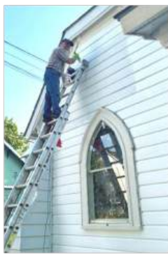
David St. Amand high atop a ladder at the northwest corner of the building.
