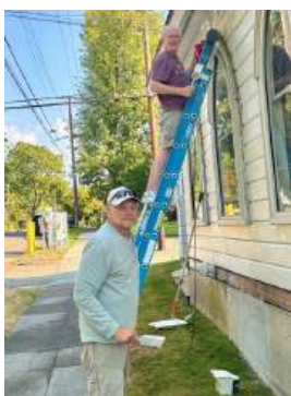
Wes Fenn & Jeff Knapp getting to work painting the west side of the building.
